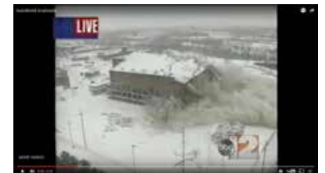
You can watch the demolition of the Flint's AutoWorld at https://goo.gl/TE1pwa .
